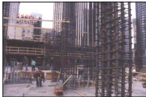
Eliminating rebar splices and reducing rebar weight at Westlake Tower, Seattle
