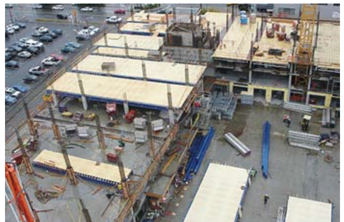
Aligned columns facilitate a clean formwork layout and maximize productivity
