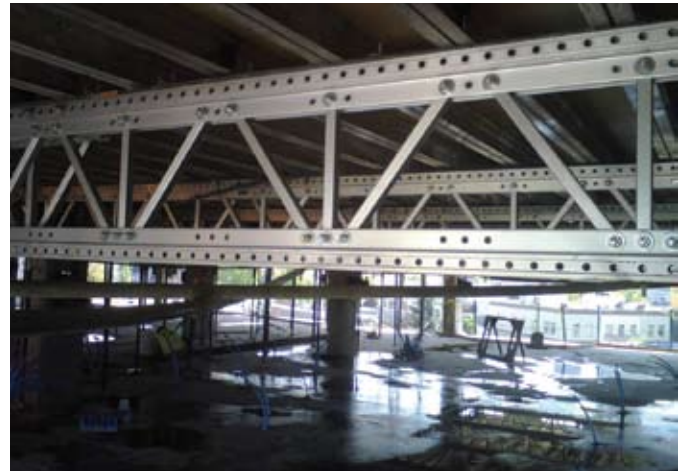
The trusses supporting these flying deck forms are fully adjustable, allowing versatility in span and spacing
